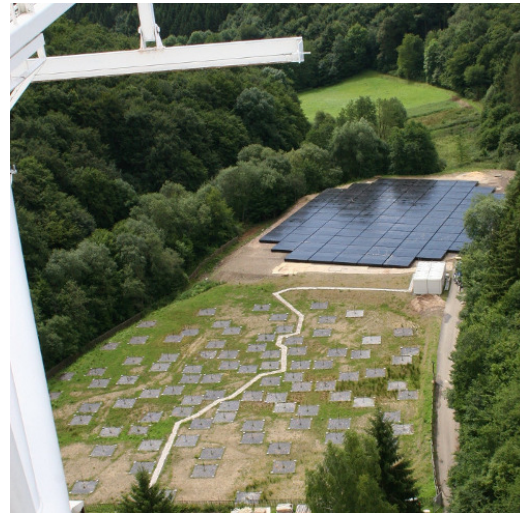
Fig. 2 International LOFAR station seen from the lower platform of the Effelsberg 100-m telescope. Front: sparse dipole array for 10–80 MHz; back: dense array of dipole “tiles” for frequencies of 110–240 MHz (copyright: James Anderson, MPIfR).
