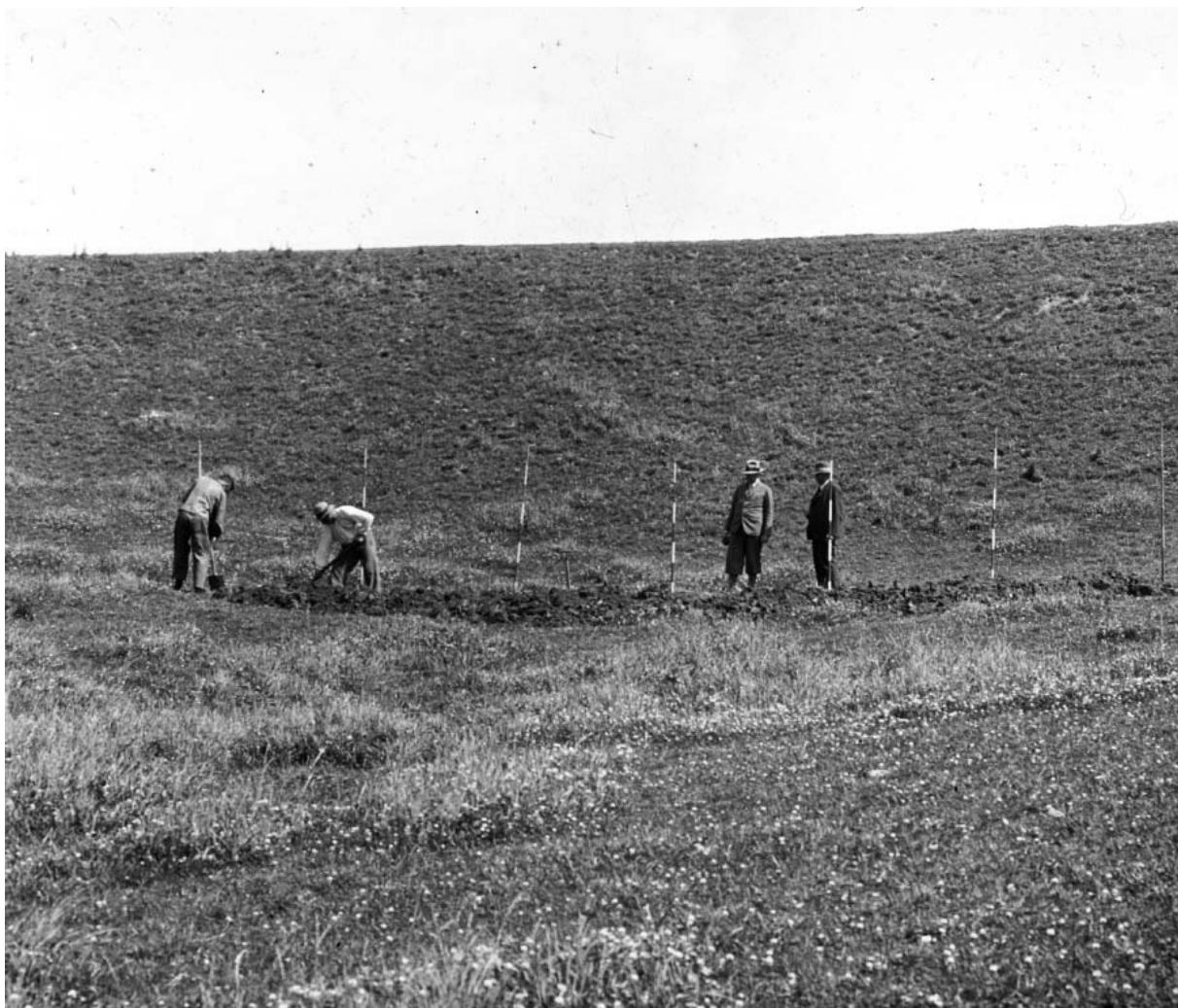
Figure 3: A photograph from the first day of the excavation: 24 July 1933. The question was whether anything at all was preserved. It was. After only a few hours of digging finds surfaced: roof tiles.
