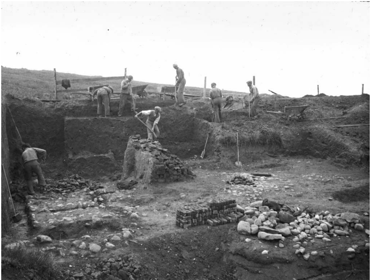
Figure 5: More expansions were necessary before the shape of the building could be seen. Here they are digging in its south-western part.
